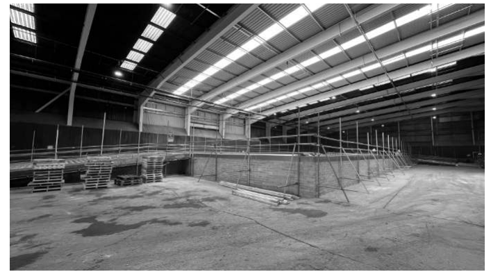
The raised platform on which visitors will park and dispose of waste.
